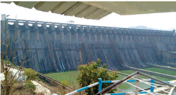
Narmada Dam - View of Spillway, Radial Gates Stilling basin
