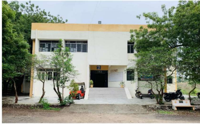
(Mechanical Workshop building)
